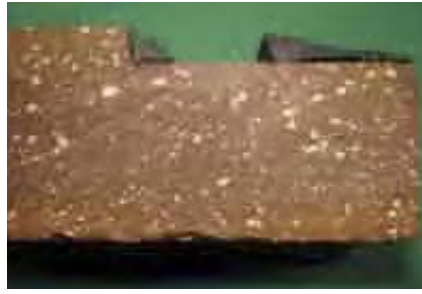
Modern day VCP pipe wall
